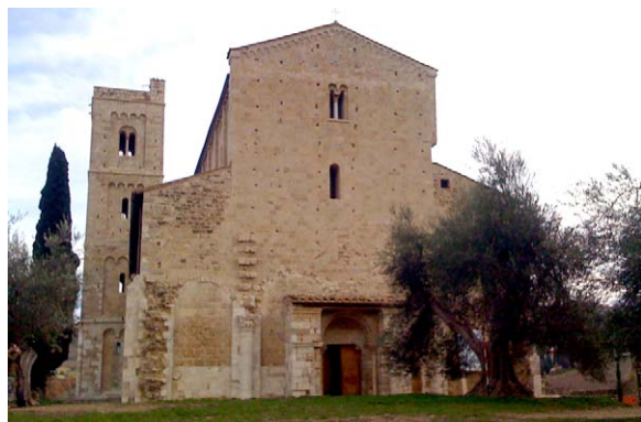
Fig. 2. St. Antimo monastery and olive trees growing close to the facade.
