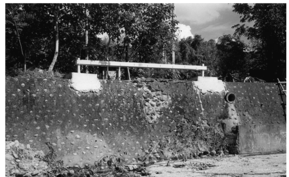
Fig. 2. (a) Schematic representation of our rod-type creepmeter [10] set up across an active fault rupturing a concrete wall. (b) Photograph of creepmeter 4 at Chinyuan.
