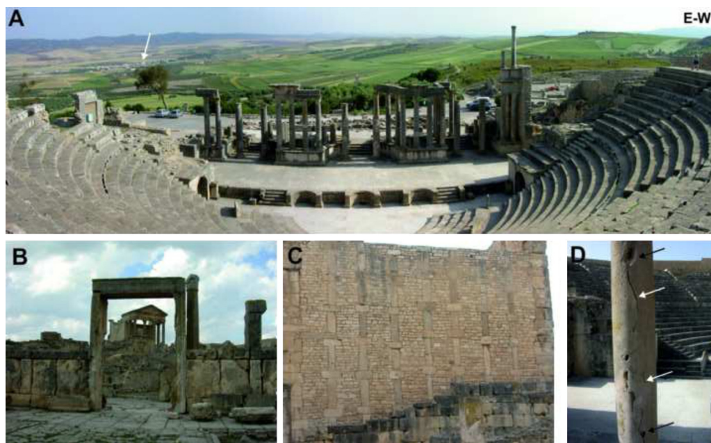
Fig. 2. Field views of some of Dougga's buildings made with nummulitic limestones. A. Panoramic view of the amphitheatre with the valley and Nouvelle Dougga (arrow) in the background (S. II AD). B. View of the market's entrance with the Capitoline Temple (s. I AD) in the background. C. Wall made of centimetre- to decimetre-sized rock blocks. Note the meter-scale blocks used in the base of the wall. D. Detail of a column from the amphitheatre showing fractures (white arrows) and macrovugs (black arrows).
