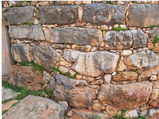
(b) Packing stones in-between larger blocks
