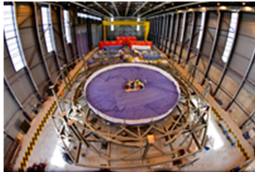
Fig. 4. A large “thermos”, the cryostat, will encase the machine and prevent heat exchanges between the ultra-cold superconducting magnet system and the environment. Procured by India, this 30-metre high, 30-metre in diameter is being assembled and welded in a dedicated workshop on the ITER site.
