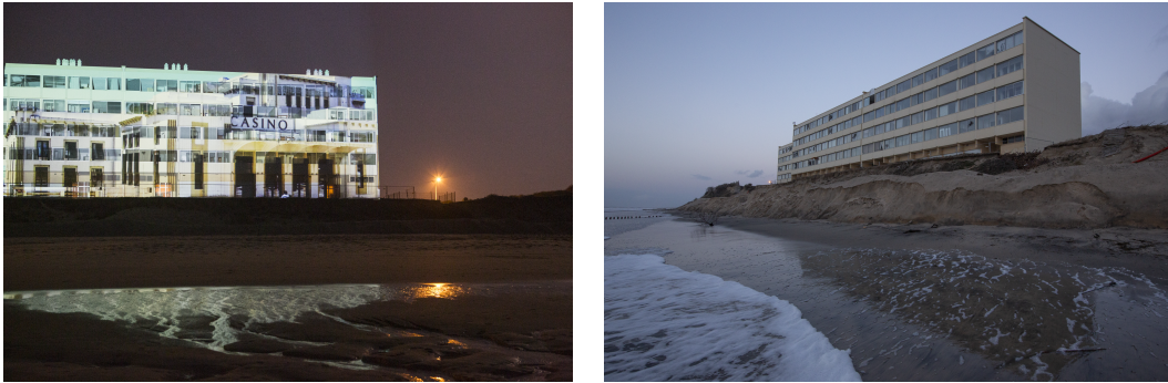
Figure 2. Photographs from an artistic perspective of Le Signal building (Soulac-sur-Mer, France). This construction, built between 1967 and 1970, was definitely abandoned in 2014 under the threat of coastal erosion and finally demolished in 2023. Credit: Le Signal@Olivier Crouzel ( https://www.oliviercrouzel.fr ).
