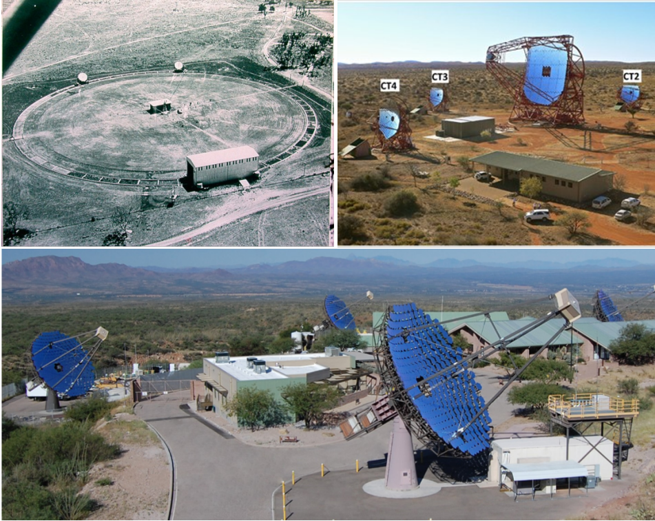
Figure 1. Pictures of different facilities used for intensity interferometry with large light collectors. Top-left: the Narrabri observatory, with two telescopes set up on railroad tracks to vary the baseline size and orientation [27]. Top-right: the H.E.S.S. site in Namibia with Cherenkov telescopes 3 and 4 specifically used for intensity interferometry [21]. Bottom: VERITAS array in Arizona with 4 Cherenkov telescopes [25].
